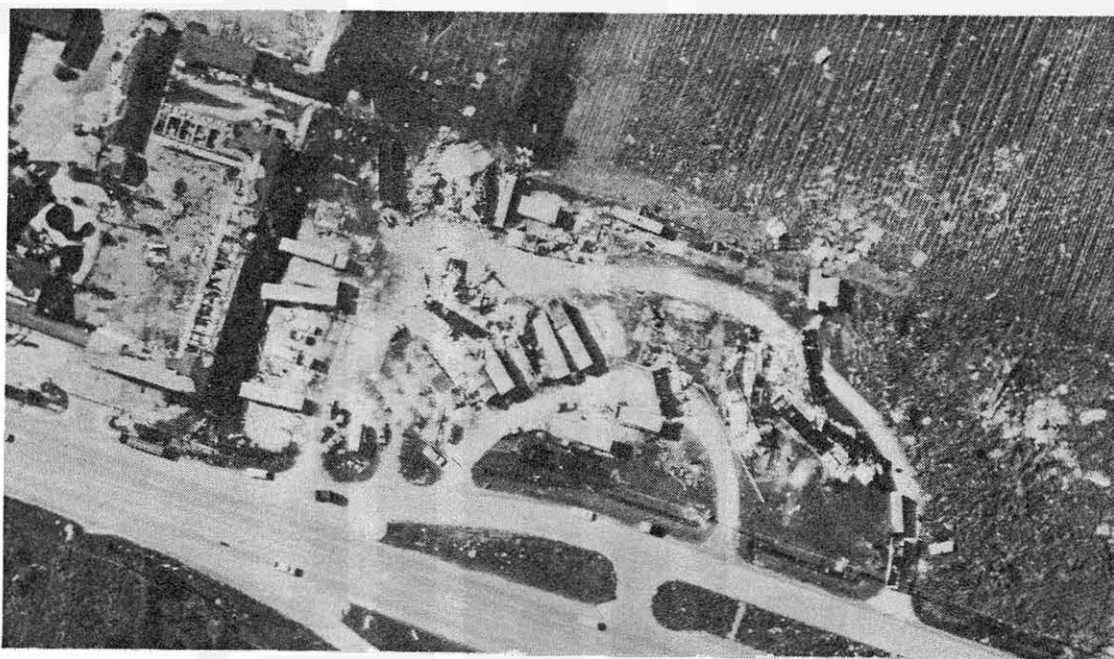
Figure 2.6 A motel and trailers west of Downtown Corpus Christi damaged by downburst winds in hurricane Celia (see Color Map No. 9). Damaging winds estimated to be upper F1 or lower F2 came from WSW. The hurricane center, to the north of the city, was moving WNW at 16 mph.
